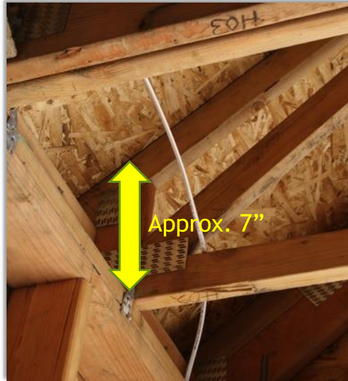
Raised Heel Truss Construction
