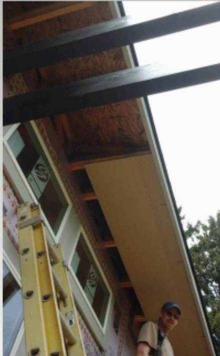
Above: Sider installing enclosed soffits, this keeps out birds and insects
