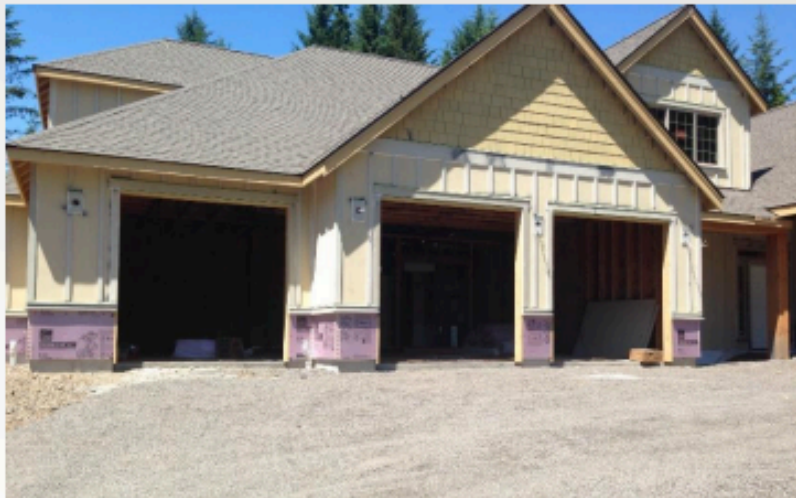
Left: House completely sided including foam underneath
